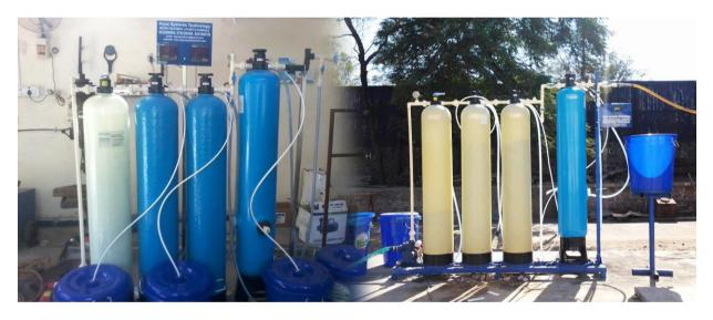
We offer completed Technical Service operators of maintenance of D.M. Plant Including Resin. The process of restoring their power or enhancing active ion concentration level is called regeneration. In this process exhausted cation and anion ions are recharged with Hydrogen (H) Hydroxyl (OH) ions.
